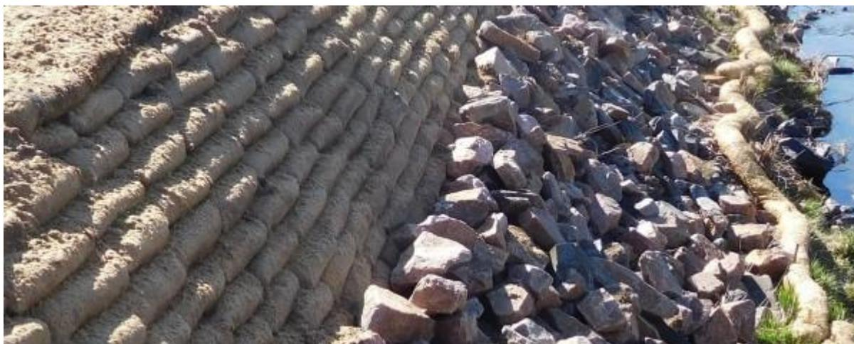
Envirolok is a Vegetated Mechanically Stabilised Earth Wall System for retaining walls, slope stabilisation, erosion control and shoreline protection.
